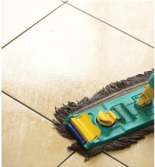
"Post-installation" cleaning helps remove residues of joint grouts, cement and lime. This operation is mandatory after installation both for glazed and unglazed tiles. Never clean tiles that are too hot (e.g. exposed to sunlight during hot summer months) since the reaction of aggressive chemicals may become harsher. In the summer, proceed with the operation during the coolest period of the day.
