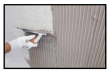
Installation of insulation panels with double buttering (on wall)
