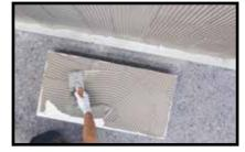
Installation of insulation panels with double buttering (back of tile)
