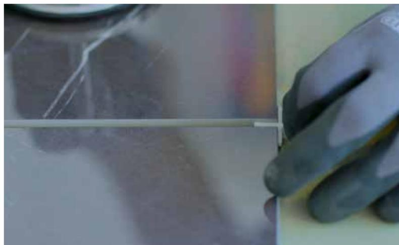
The use of 2mm spacers, which can be easily purchased, makes it possible and very simple to create uniform grout lines. The spacers will not be removed, but will rather be covered by the grout, so be sure to push them far enough down.
