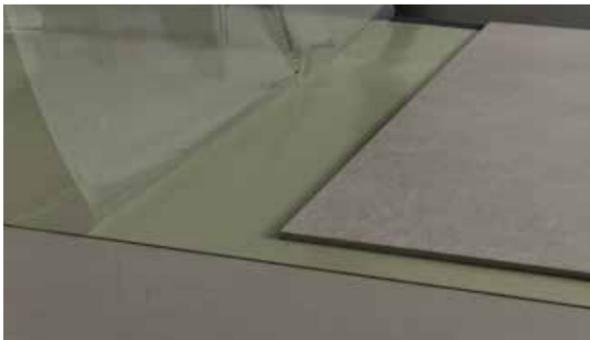
DO NOT remove completely the protective film. The film must be removed gradually while the Slimtech Plus slabs are being laid.
